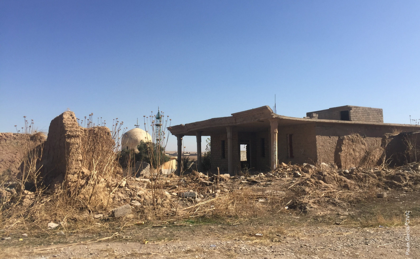
October 2019, Balad, Salah al-Din, Iraq: An unfinished building.
