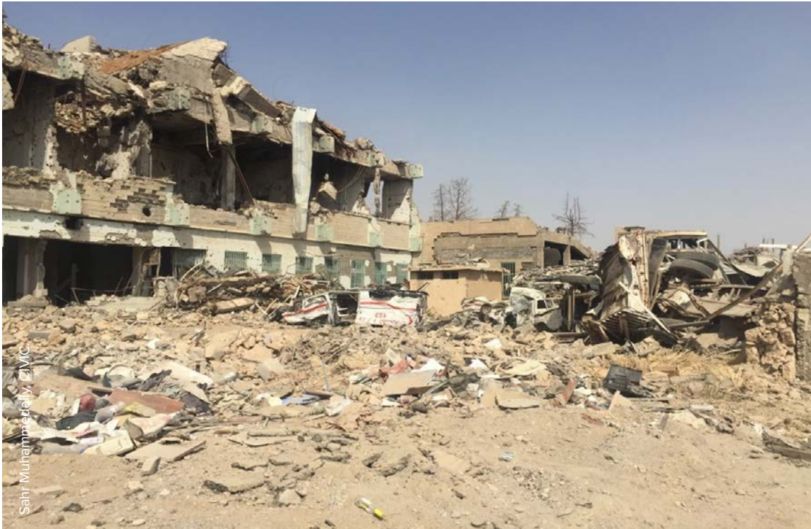
August 2017: Hospital in West Mosul rigged with IEDs and destroyed.
