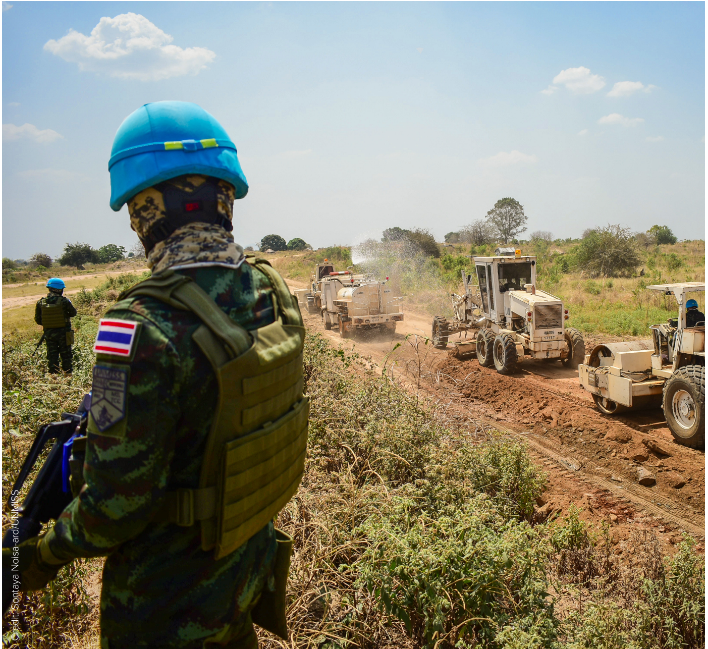
November 20, 2021, Juba, South Sudan: UNMISS engineers repair a 155-km main supply route linking South Sudan's capital, Juba, to Yei. The objective was to boost trade and allow communities to convene and have access to necessary services.
